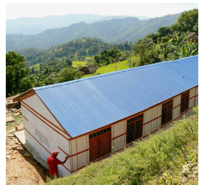
Local builders working with Smart Shelter on a stone and rubble school in Nepal. Horizontal bands are used to tie the structure together in a way that resists collapse. The methods are indicated on completed building. Images: Martijn Schildkamp / Smart Shelter Foundation
