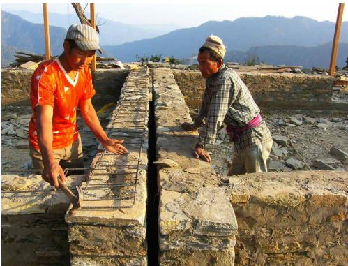
Local builders working with Smart Shelter on a stone and rubble school in Nepal. Horizontal bands are used to tie the structure together in a way that resists collapse. The methods are indicated on completed building. Images: Martijn Schildkamp / Smart Shelter Foundation
